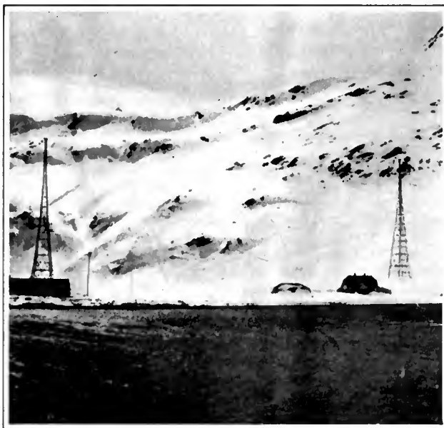
MARCONI'S NEW 6-KW, 2000-METER TRANSMITTER This wireless telegraph station at Grytviiken, South Georgia, maintains a daily telegraph service with the Falkland Islands which in turn communicate with Montevideo
